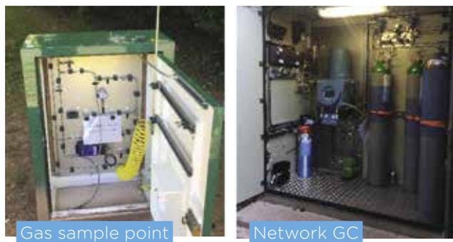
**Figure 14: Network monitoring facilities**
