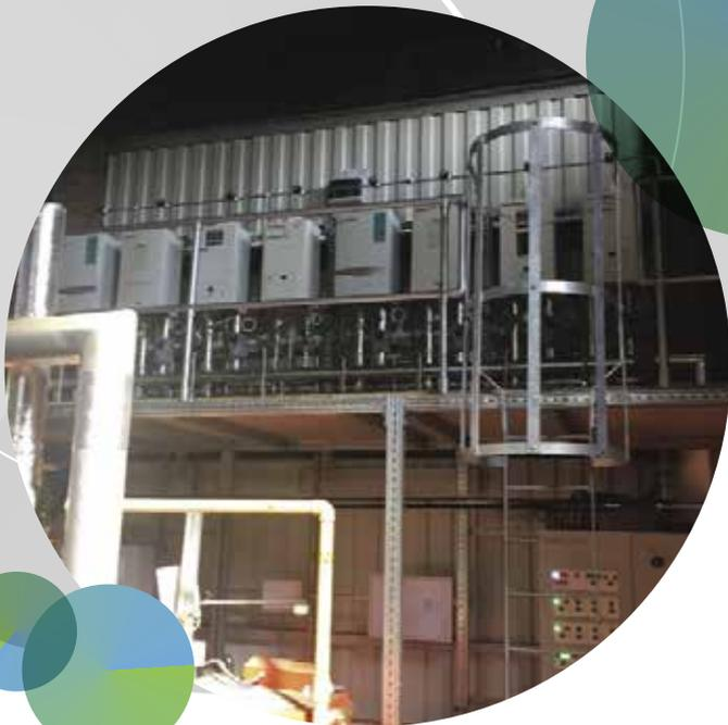
**Figure 23: Full boiler installation**
