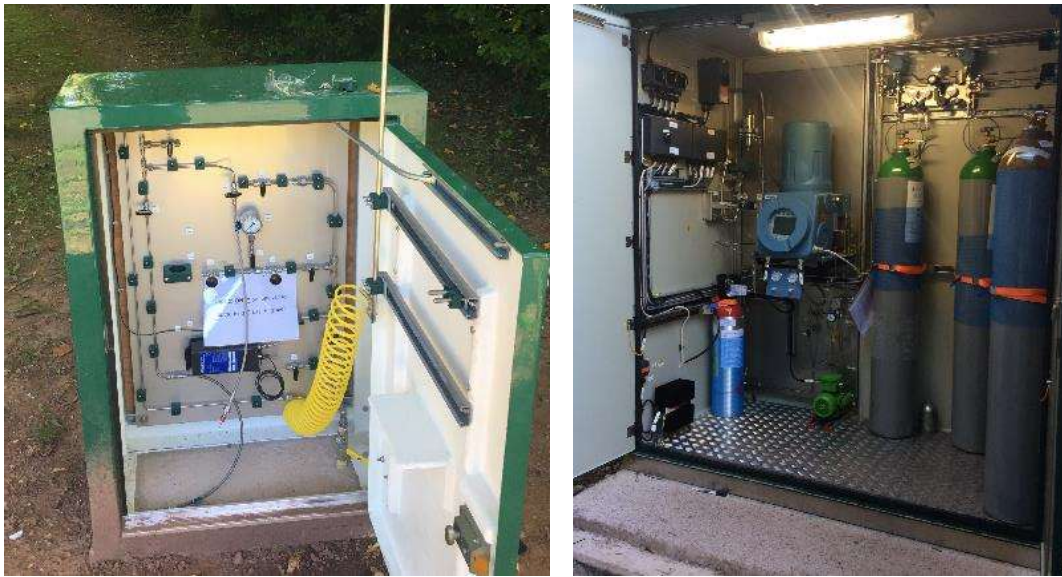
Figure 13: Gas sample point (left) and Network GC (right)
