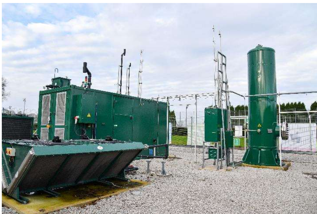
Figure 10: Installed electrolyser system
