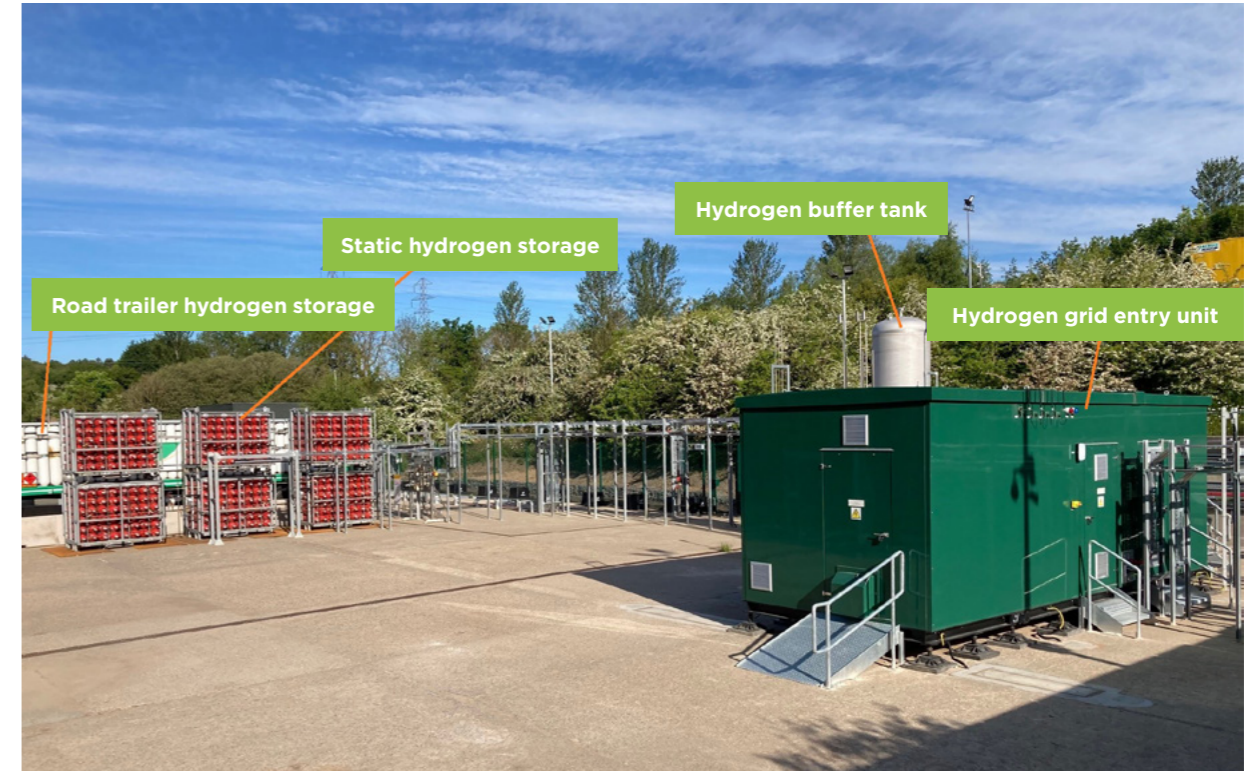
Figure 12: Image of Low Thornley compound highlighting various assets.
